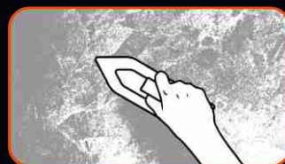
phase III: If needed, apply second coat similarly to the previous one.
