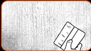
phase V: Coat the surface with Decorative Varnish (colourless).
